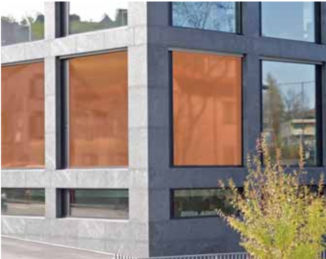
Head Office of Sefar AG, Heiden, Switzerland. Glass facades with SEFAR® Architecture Vision fabric CU 140/50, single-side coated
